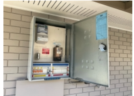
Showing example of the property/conditions at the time of the inspection
