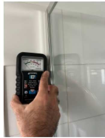
Showing examples of moisture meter readings taken on site, where the level recorded did not show an elevated reading.
