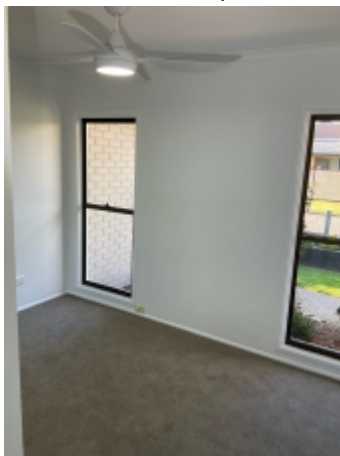
Showing example of the property/conditions at the time of the inspection
