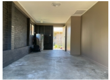
Showing example of the property/conditions at the time of the inspection
