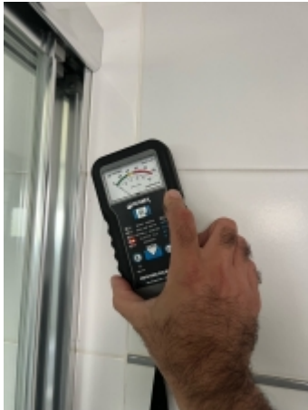
Showing examples of moisture meter readings taken on site, where the level recorded did not show an elevated reading.
